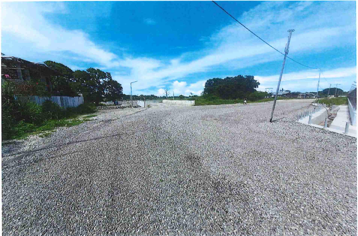
Figure 33. External road down to NSC land – Complete tar sealed
