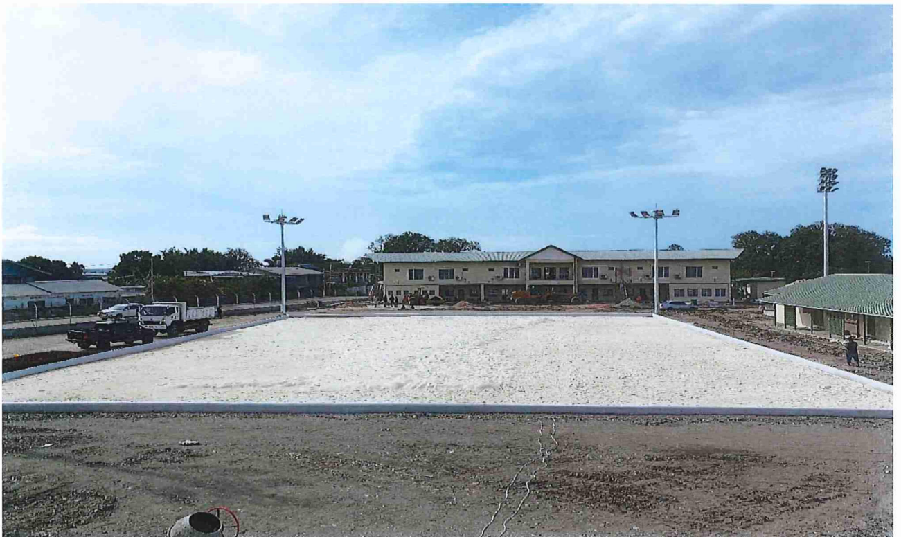
Figure 23. View @ Admin Building
