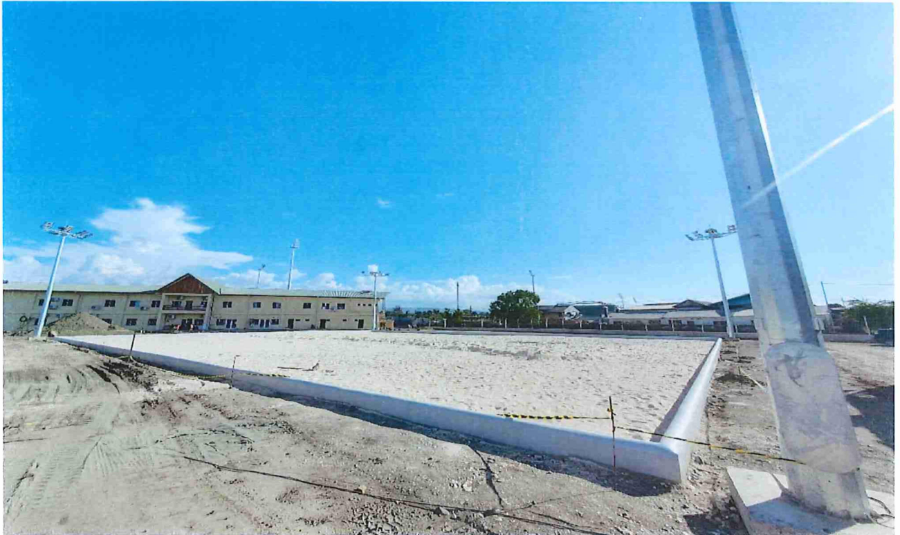
Figure 22. First load white sand filled in (200cubic)
