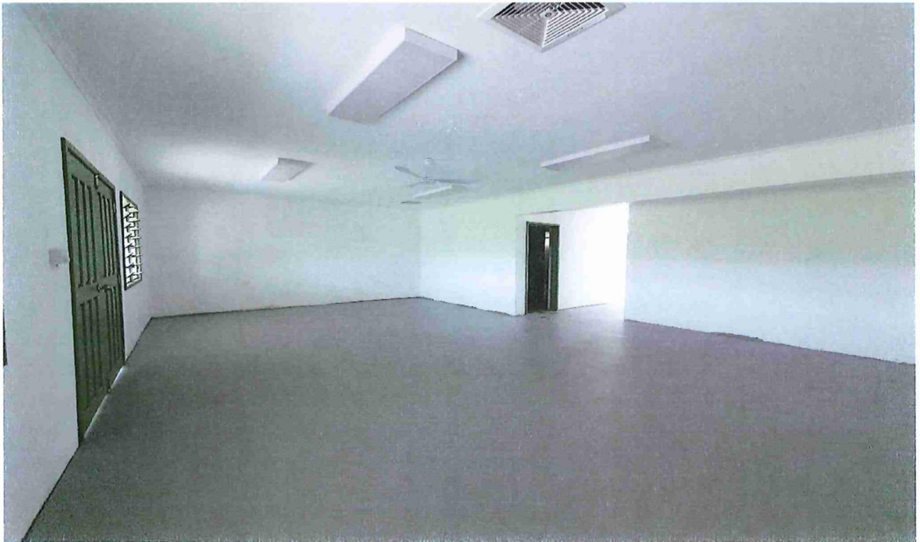
Figure 12. Referee chamber –vinyl flooring finishing
