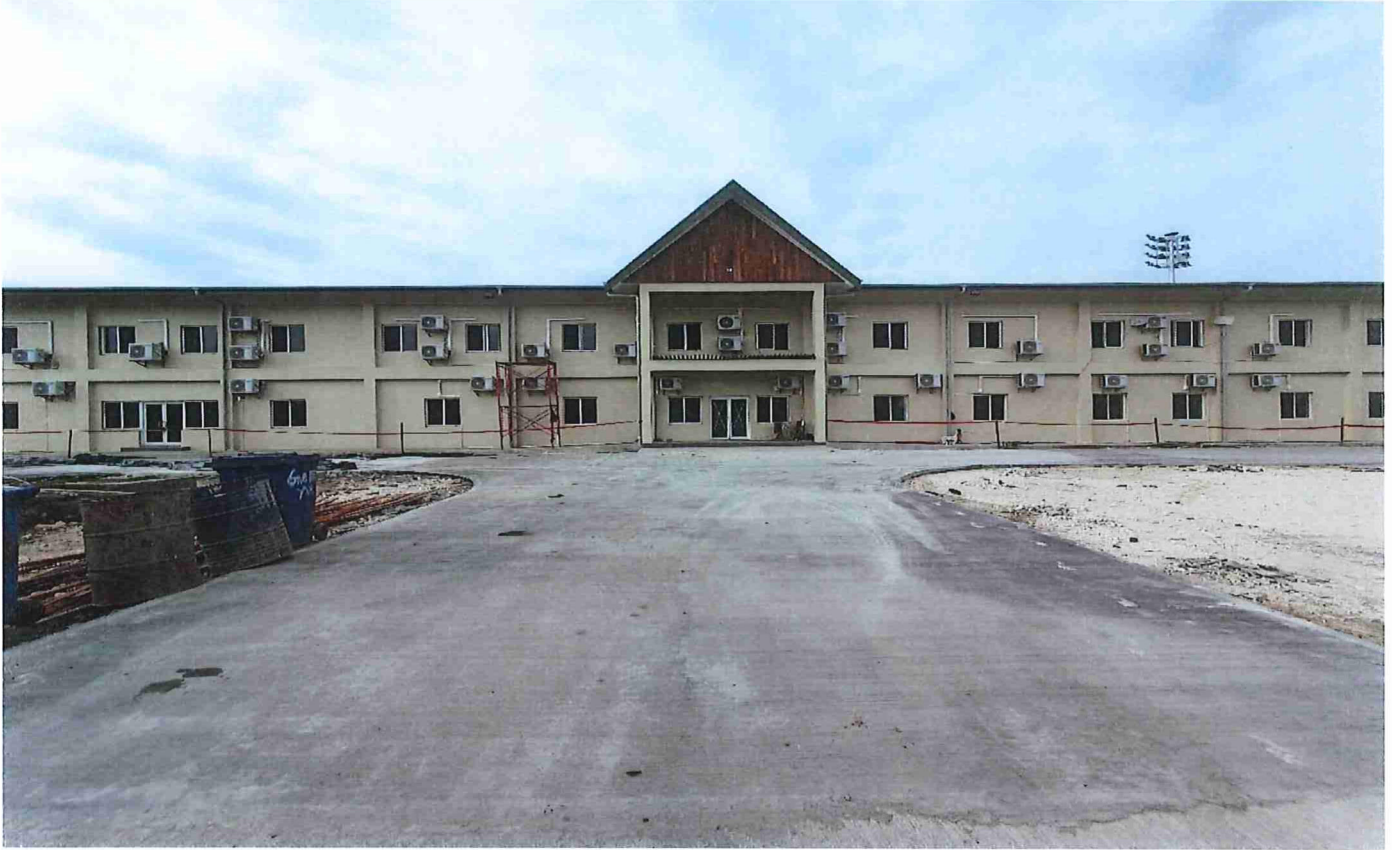
Figure 1. Front view @main entrance
