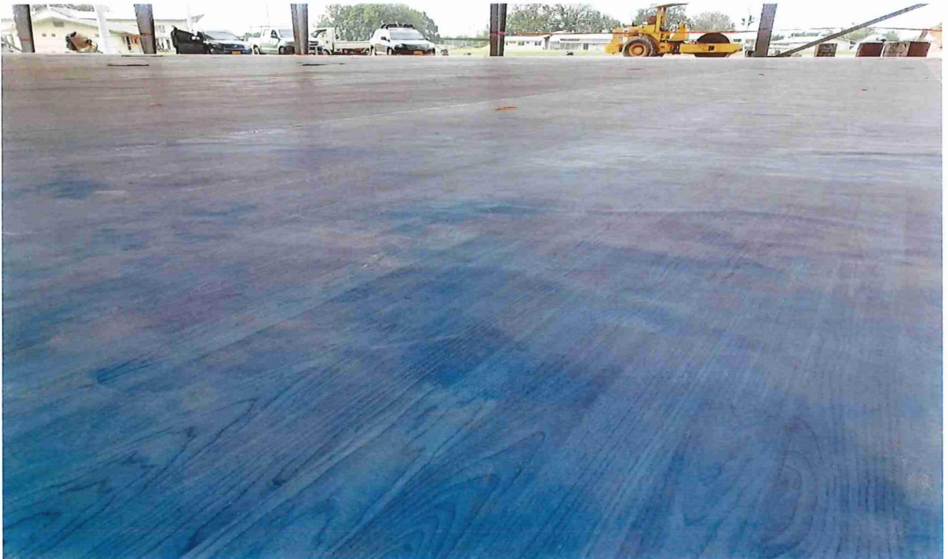
Figure 15. Lumps on vinyl mat surface – cause uneven surface – issue has already been addressed
