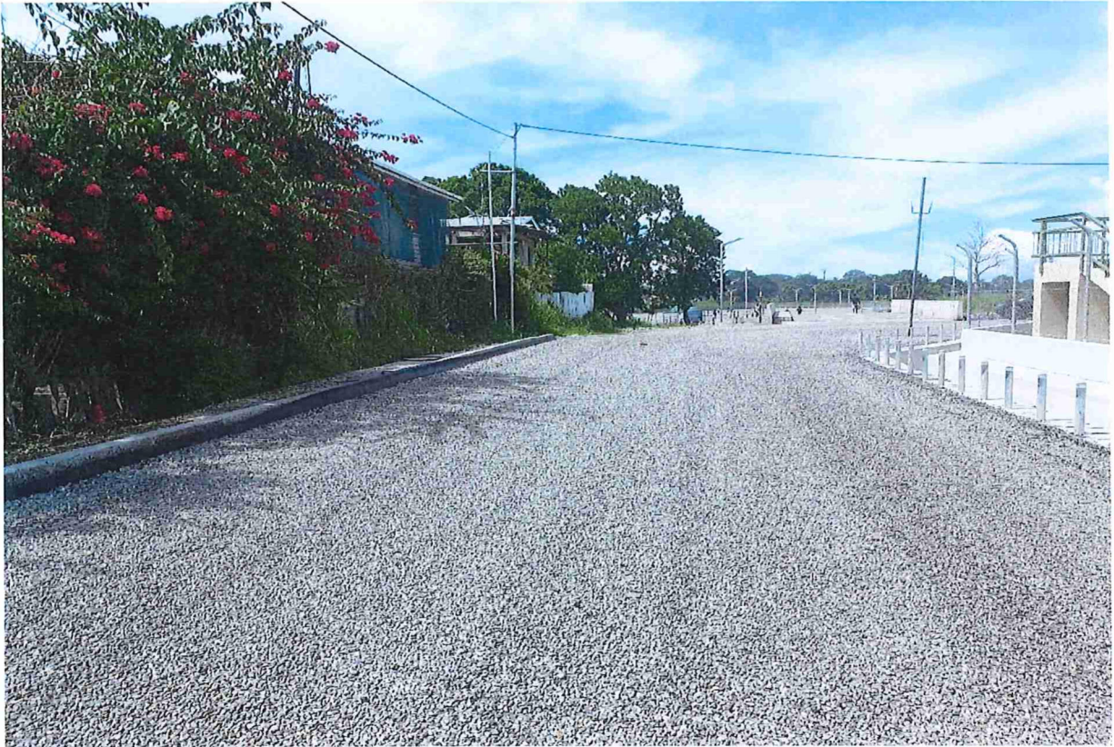
Figure 32. External road down to NSC land – Complete tar sealed
