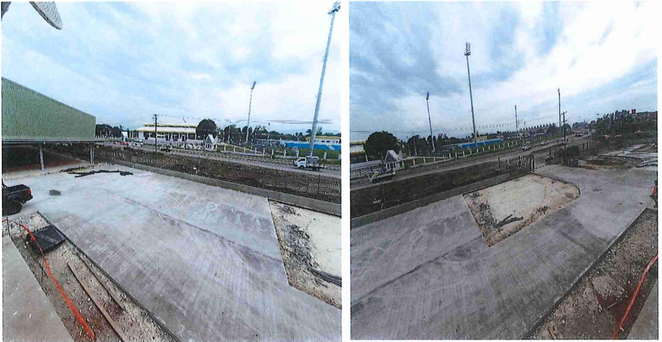
Figure 27& 28. Concrete slab carpark
