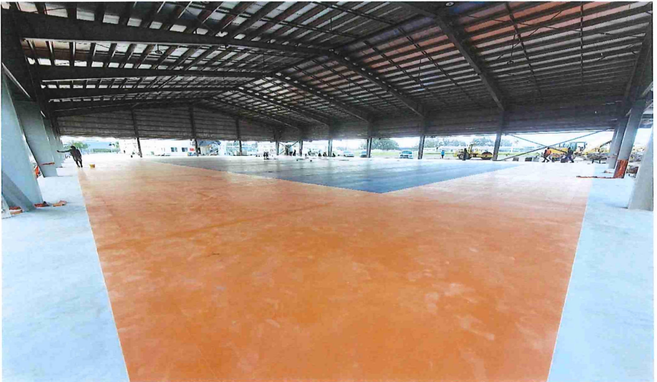
Figure 14. Complete installation of vinyl mat flooring (4.5mm thickness)
