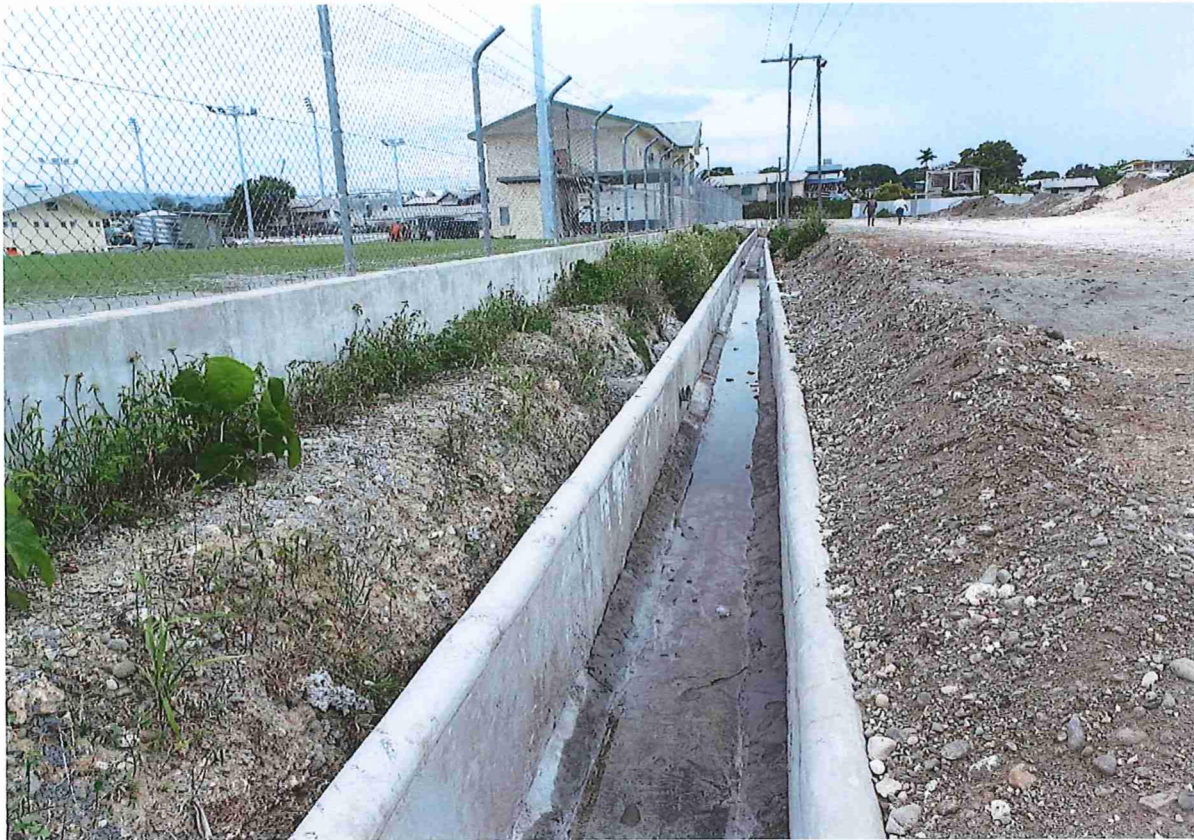
Figure 30. Storm water drainage (North end) – complete cement rendering
