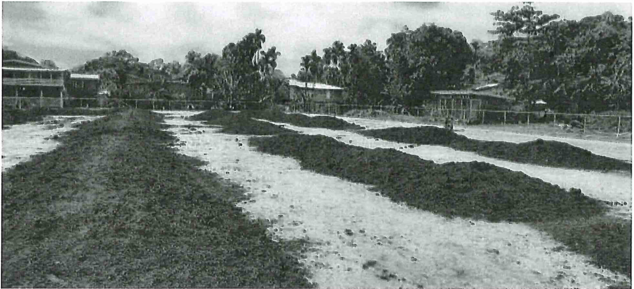
White River Field. (Top soil ready for spreading and compaction)
