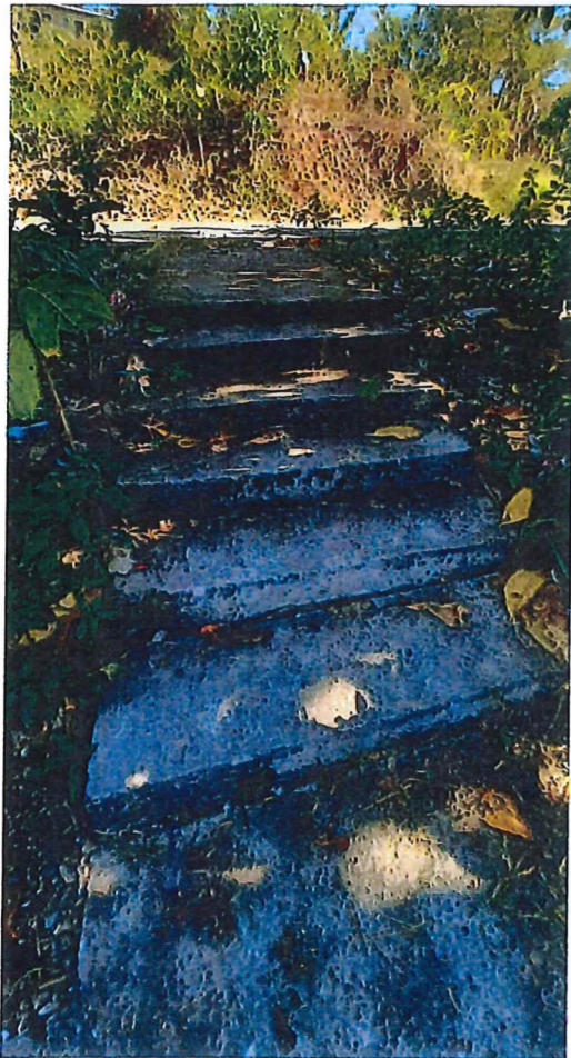
Figure 12 and 13: Ramp for demolition, cleared and disposed to proposed site.
