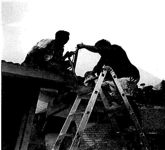
*Mounting entry box for service line to attached.
