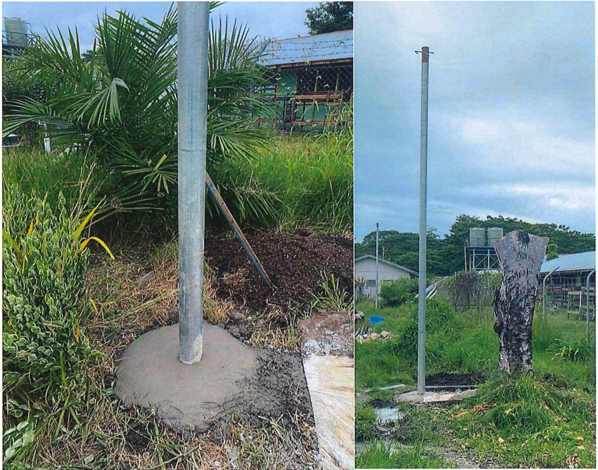
Figure 1 New service line poles installed for supply connection to building 7,8,9 & 10.
