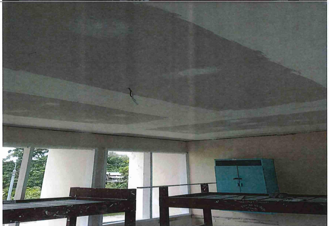
Top floor Fibro ceiling and three coat gyprock compund
