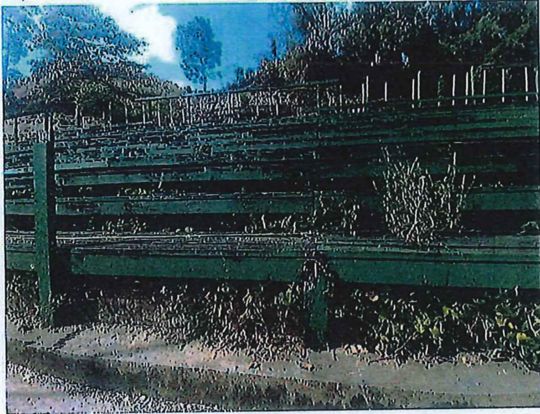
Figure 7: Southeast Stands – Front View
