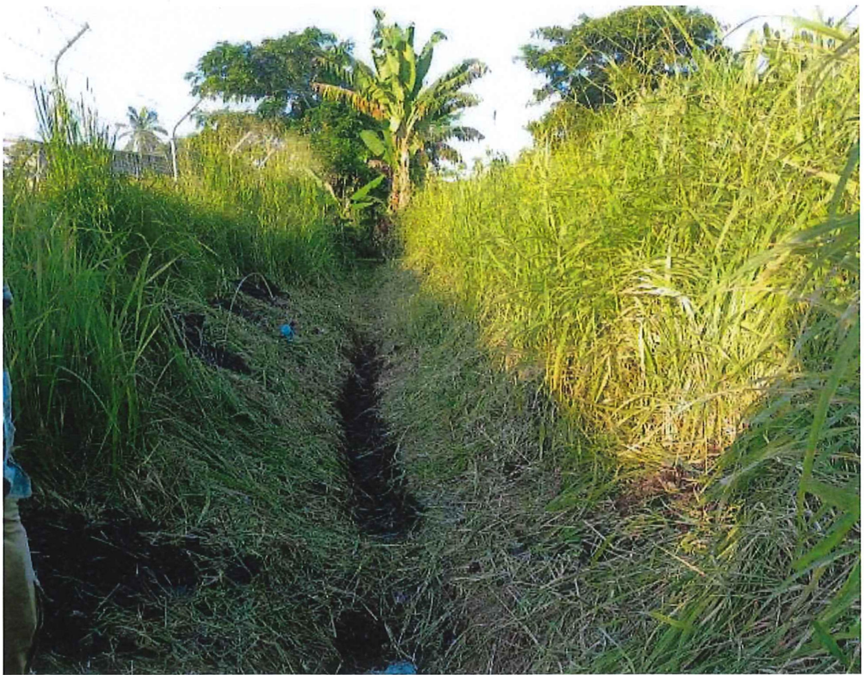
Figures 3, 4 and 5. Cleared existing ditch for Topography Survey
