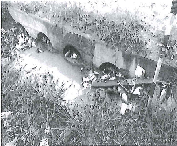
Figure 1- Existing Culvert at Chainage 678.53 along the main road
