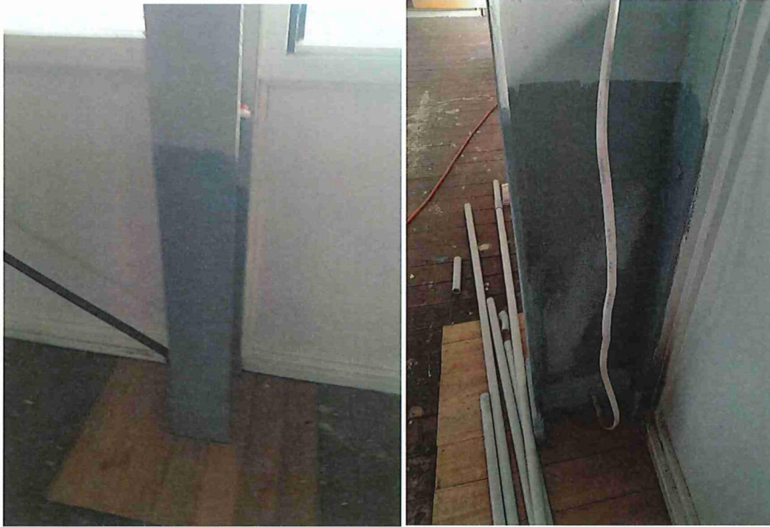
Photos of restrengthening of steel columns
