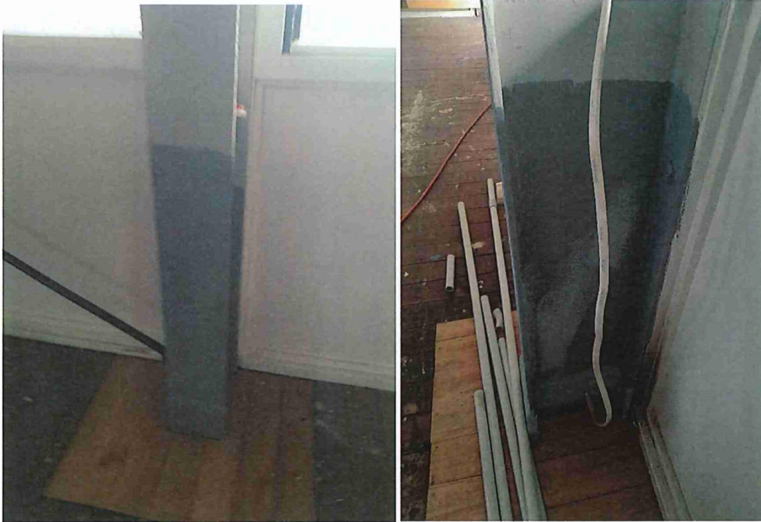
Photos of restrengthening of steel columns
